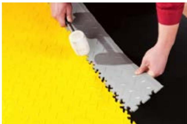
Generally there is no need to secure the Motolock ramps unless it will be exposed to prolonged direct sunlight, which may cause the ramps to become displaced as it softens we would suggest that you glue down using a high temperature contact adhesive. The ramps lock in line with each tile.
