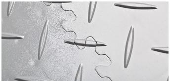
Please do not force the tiles together, offer up the corner of the tiles and using the non-marking rubber mallet tap the joints together gently, if tiles are not locking together without a lot of force then they may not be properly aligned or you are doing something wrong.
